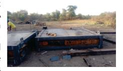
layers laid parallel and perpendicular to the track alternatively. The weight of the composite structure works out to 9 to 10 MT per bearing. C – Bar or tie bar of 6 mm dia tied to bind 2 sleepers together. Manufacturing of the structure can be done at site or in workshops and thus, higher quality can be maintained. Speed is
