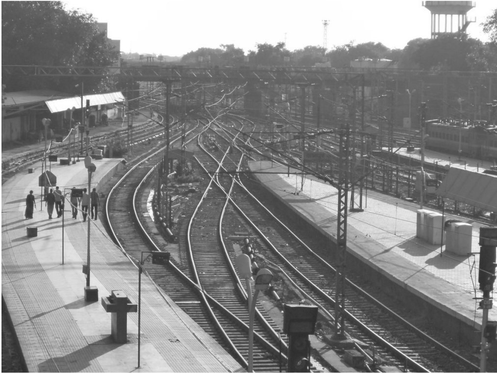
Fig.3: Cross over from platform 1 with diamonds along PF 2 & 3 for connectivity to 3 rd and 4 th lines
