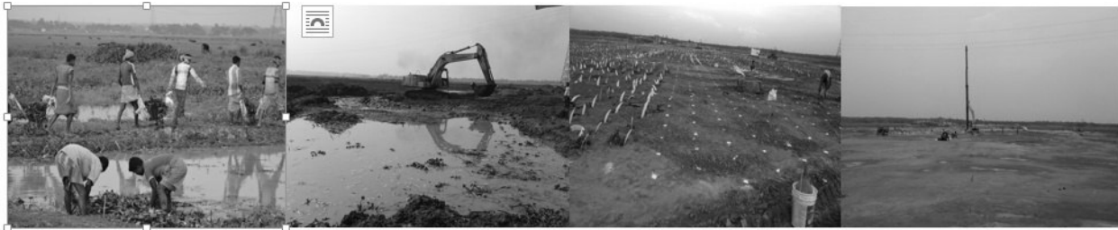
Fig. 4: Site Clearance & Levelling, Marking of Points & Installation of PVDs
