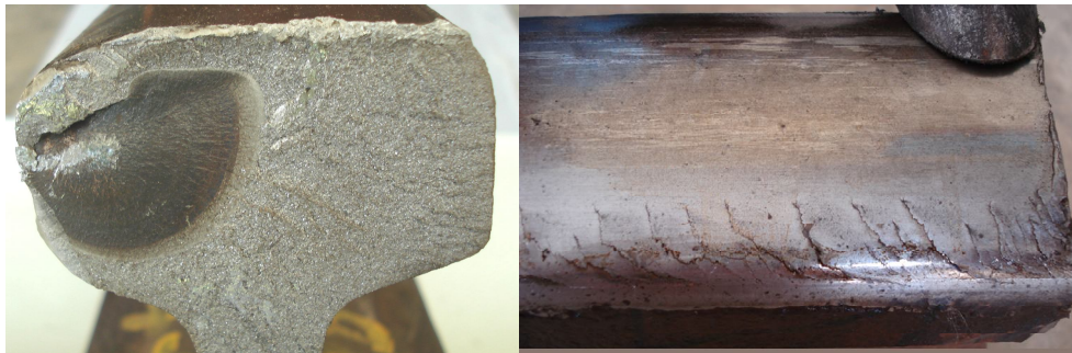
Plate1, 2: Transverse Defect in UIC 60, 880 Grade Rail covering 30% of railhead area leading to derailment at New Faridabad Station in April 09. Nucleus of fracture initiation corresponds to landing of shear crack present on gauge side of rail table. Adjoining Plate shows extent of Head Checks at the location. Question: Did head checks mask defect?
