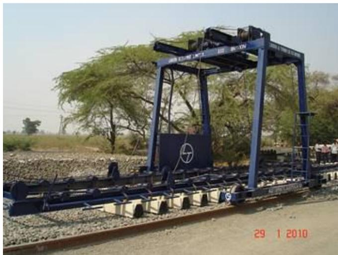
This portal may lift 15-20 sleepers in one round and move to the location where these are to be laid. After reaching to the location sleepers are released on formation or ballast bed and portal moves back to bring more sleepers. By this process only sleepers are laid initially and after completion of sleeper laying, rails available as auxiliary track are moved inward and fixed on sleepers. Hence by this process double handling of rail is avoided. Since in this
