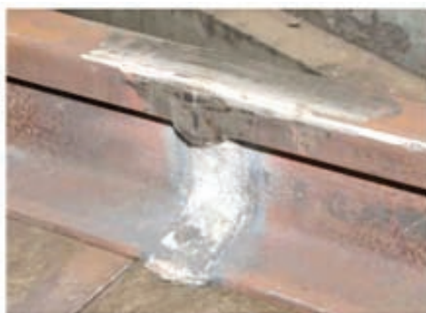
Fig.2.7 Finished weld
