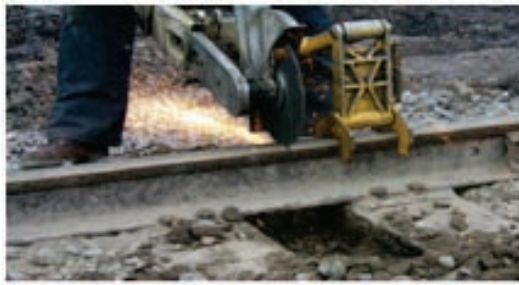
Fig. 1.2 Abrasive disc cutter
