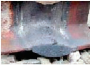
Fig. 6.1 Combination joint
