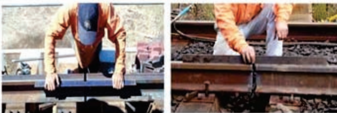
Fig.1.5 Checking alignment with straight edge
