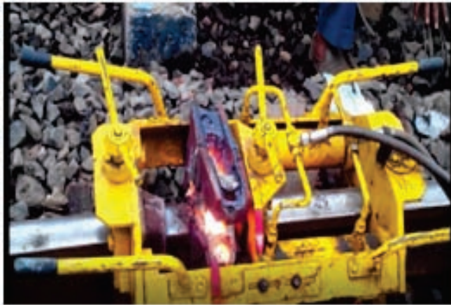
Fig. 2.4 Weld Trimming Operation
