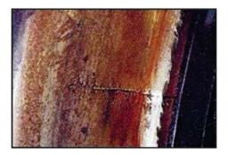
Fig.3.17 Thermal Cracks
