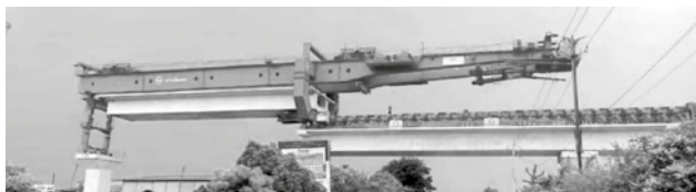
Figure 19: Erection of Full Span Girder by LG (Source: HSR Site Photo)
