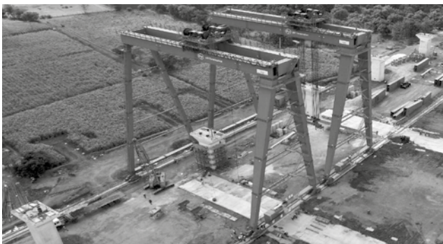
Figure 10: Bridge Gantry (Source: HSR Site Photo)
