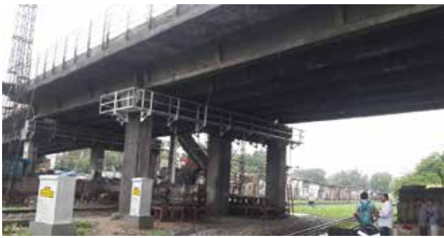
Figure 1 Road Over Bridge at Pratapnagar, Vadodara
