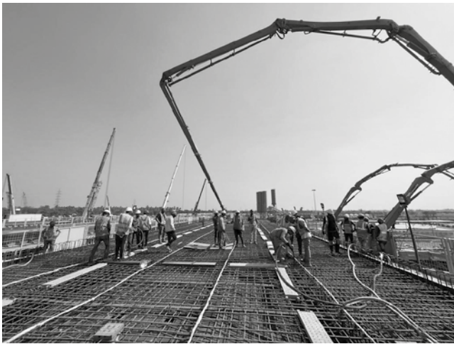
Figure 7: Casting of full span girder (Source: HSR Site Photo)
