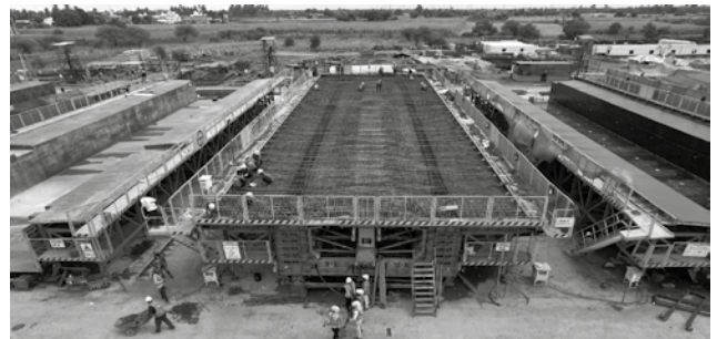
Figure 6: Sliding of Inner Mould (Source: HSR Site Photo)
