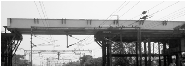
Fig.1 : Erection of a composite girder over electrified railway tracks
