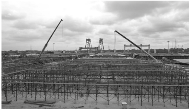
Figure 4: Tying of Rebar Cage ( Source: HSR Site Photo)
