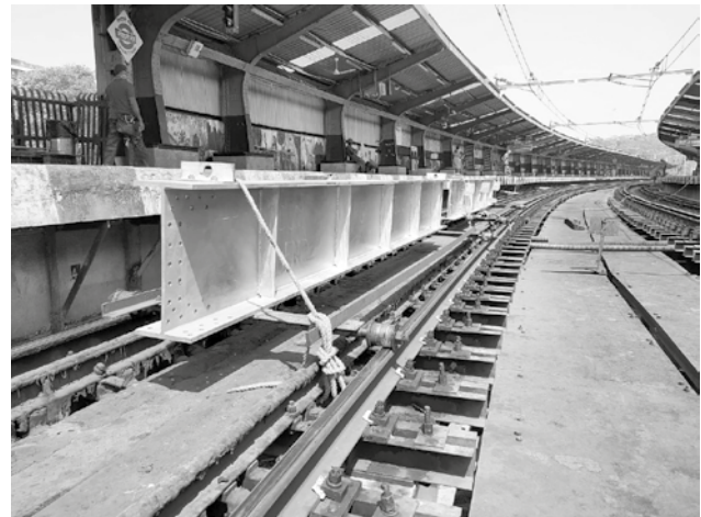
Loading of Newly fabricated upon Dip-Lorry @ Wadibunder Yard
