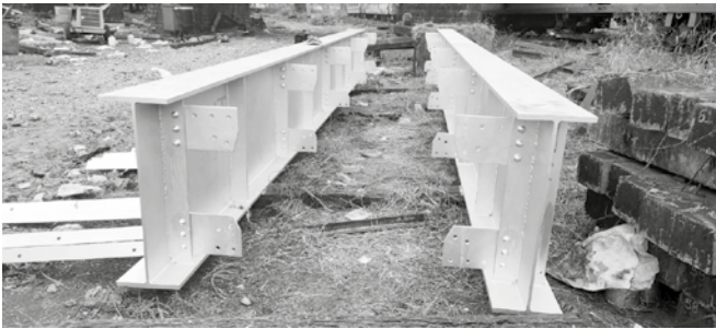
Newly fabricated Girders placed at Wadibunder Yard
