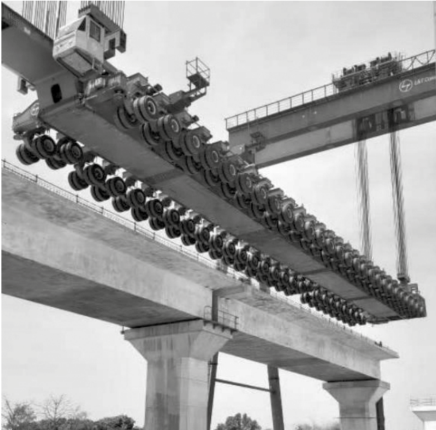
Figure 12: Girder Transporter (Source: HSR Site Photo) [8]
