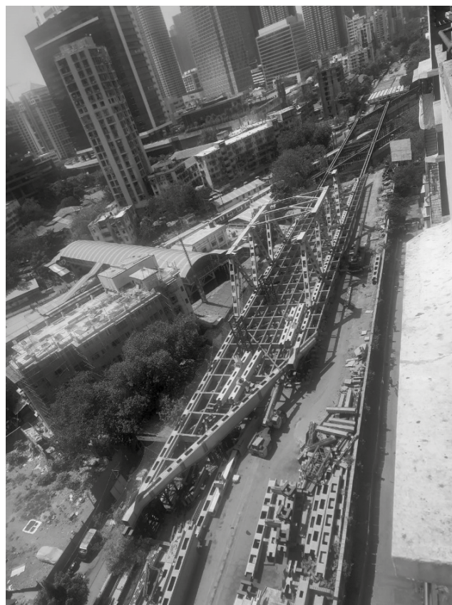
Fig: Trestle arrangement and Girder erection in progress
