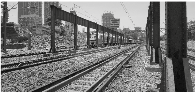
Fig: Retained substructure as temporary intermediate support
