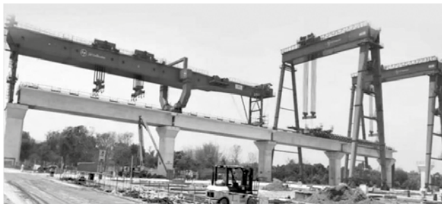
Figure 17: Erection of LG and GT (Source: HSR Site Photo)
