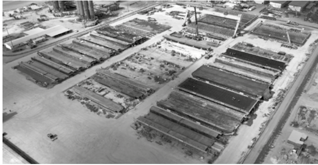
Figure 3: Assembling of Moulds (Source: HSR Site Photo)
