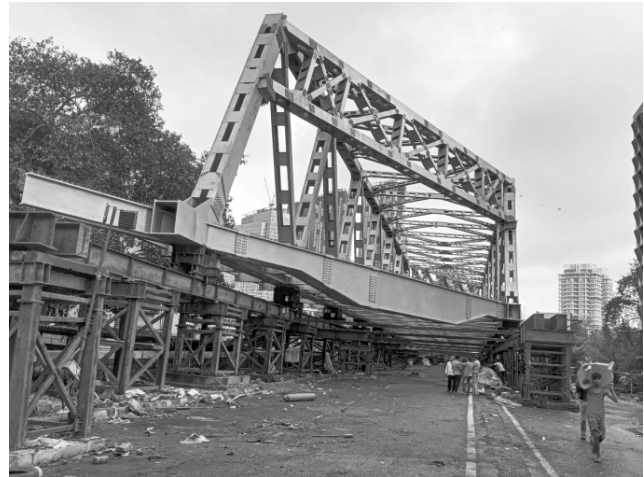
Fig: Assembly of OWG in retained approach road
