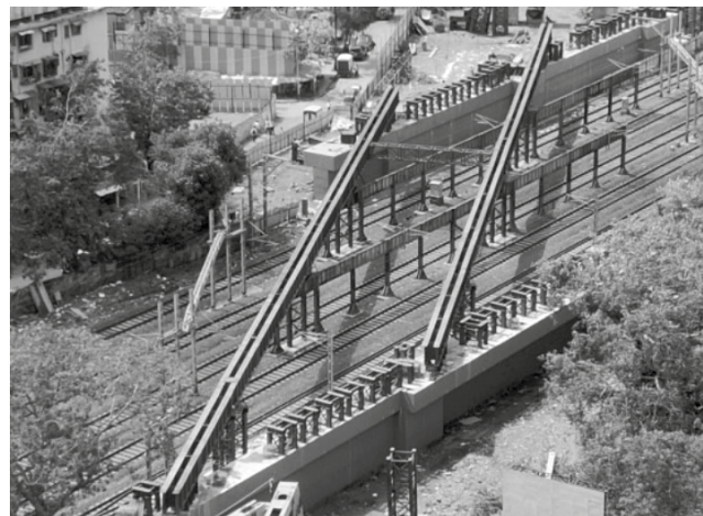
Fig: Temporary girders launched and resting on retained structure
