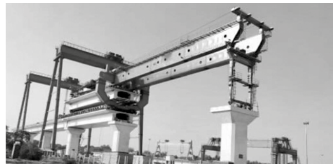
Figure 11: Launcher ( Source: HSR Site Photo)
