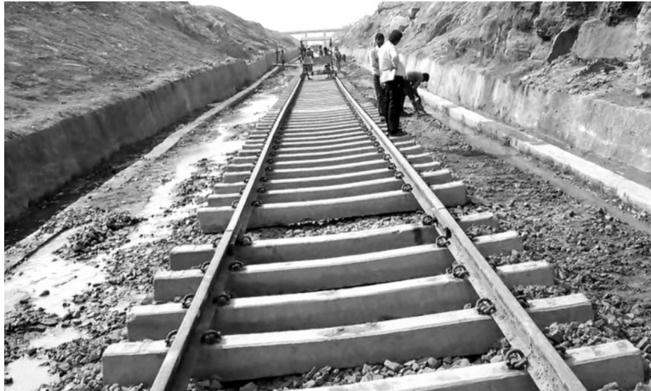
Side drain- higher than formation level
