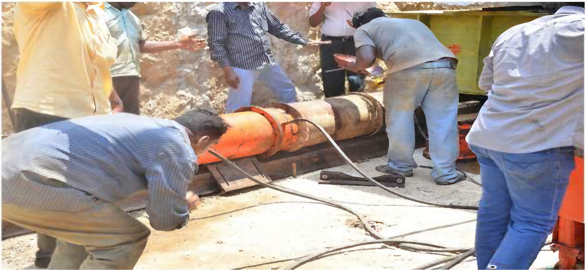
Further Pushing using the spacers
