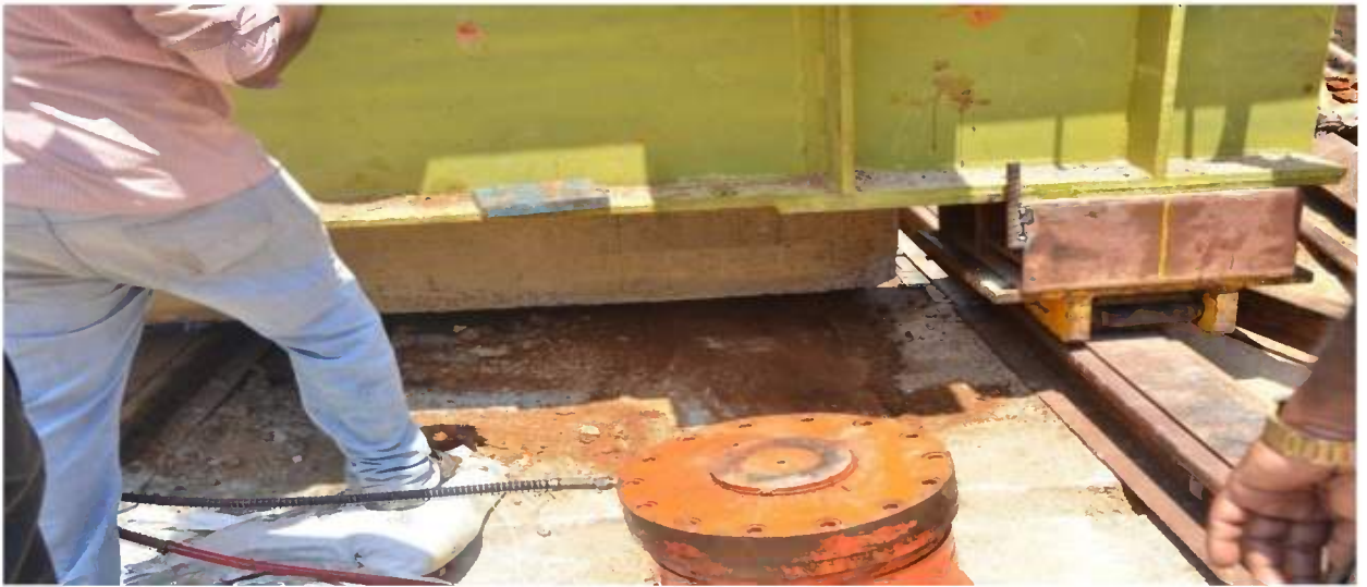
Rolling arrangements in front of RC box
