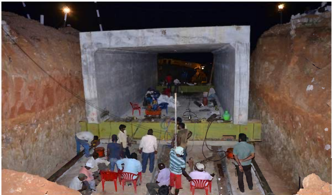
Pushing in progress
