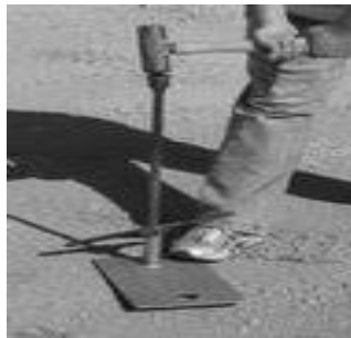
Fig. 3 : Site preparation Device with Drive Pin and Hammer etc.
