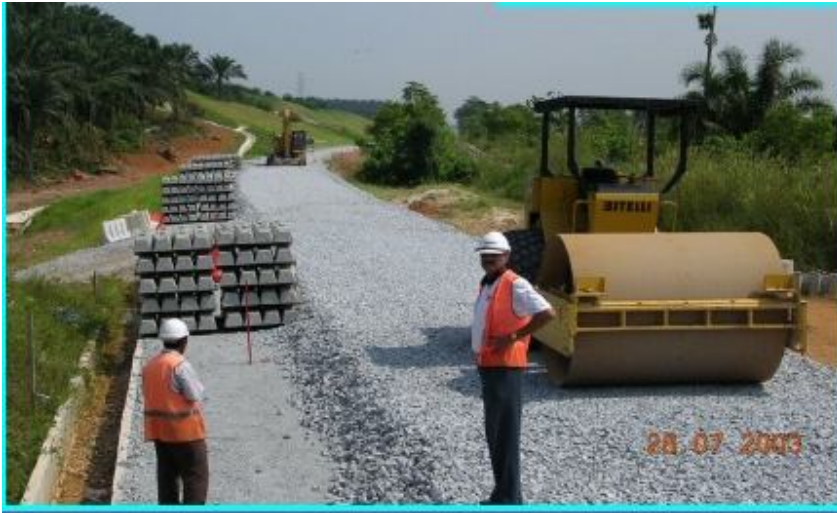
Fig. 5 – Roller compacting the Ballast
