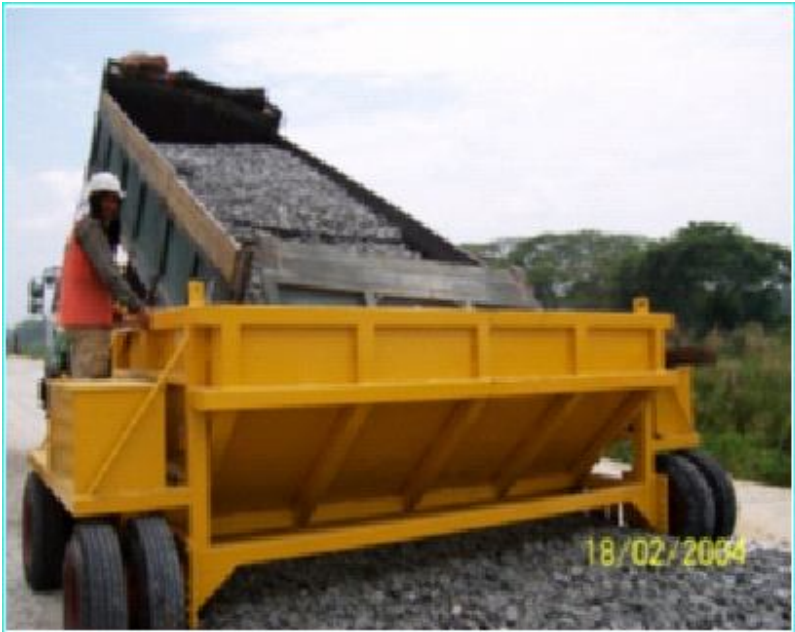
Fig. 3 - Ballast Distribution Hopper
