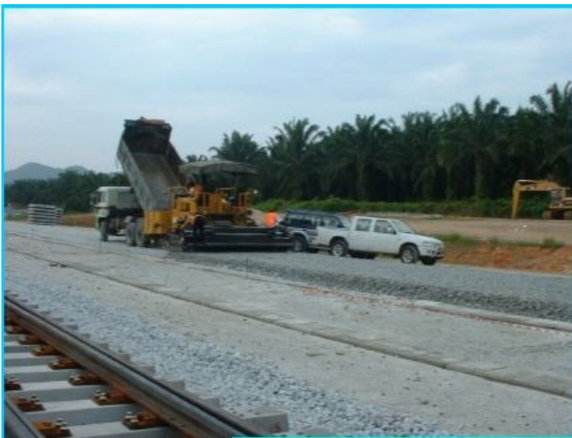
Fig. 4 – Grader for leveling the Ballast
