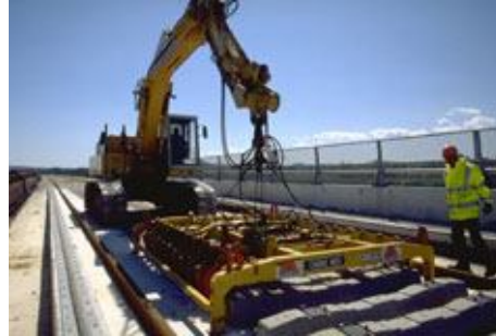
Laying alternate sleepers with the lifting beam
