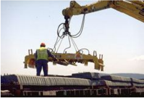
Sleeper lifting beam Discharging Sleepers onto the platform
