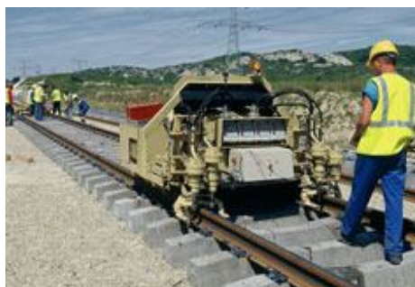
Machine for installing rail fastenings on the sleepers
