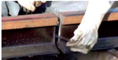
Fig. 4.2: Adjusting the initial gap
