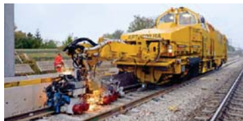
Fig. 3.2 : Flash butt welding by mobile unit
