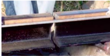
Fig. 4.3: Alignment of the rails
