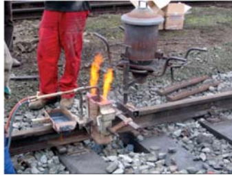
Fig. 4.6: Pre-heating of the rail ends
