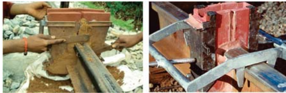
Fig. 4.4: Fixing of moulds and mould shoes
