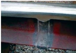
Fig. 4.10: Finished weld
