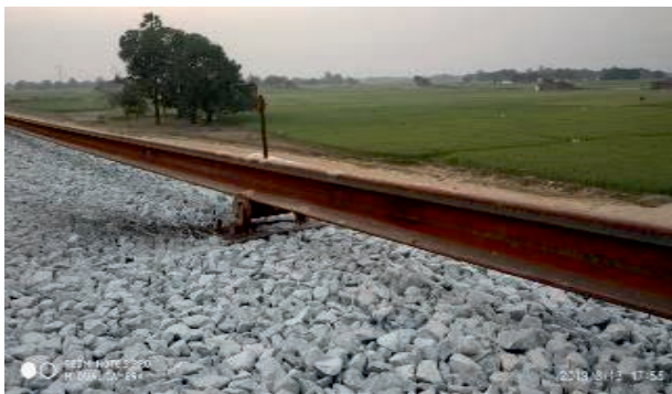
Fig. 7.17 Unloaded Rails on Rollers
