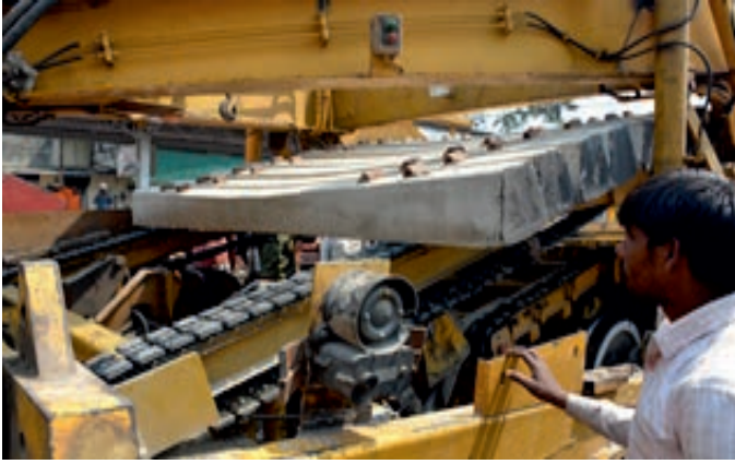
Fig. 5.9 Sleeper Feeding during Working
