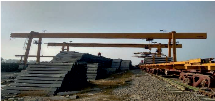
Fig. 7.5 Loading of Sleepers on BLCA Wagon.
