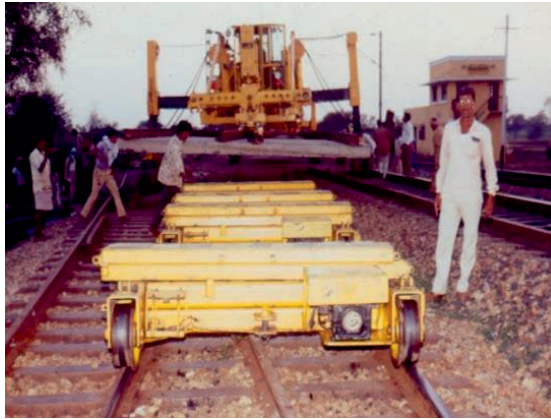
Fig. 6.8 Trolleys being Released
