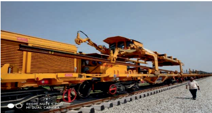
Fig. 7.13 Pulling of Rails from BLCA Wagon
