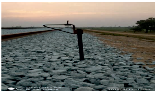
Fig. 7.9 Reference Peg for Alignment
