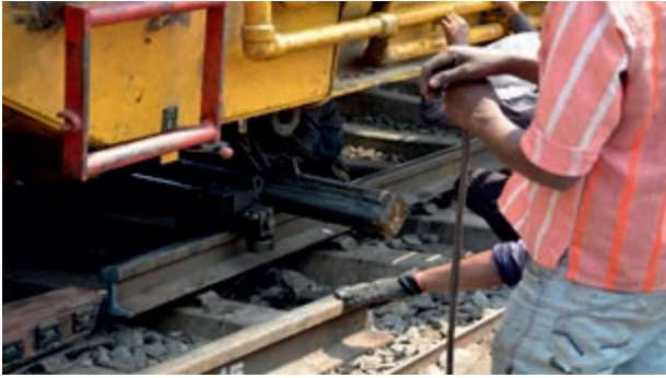
Fig. 5.5 The Rail being Slew Out
