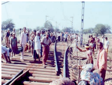
Fig. 6. 6 Dismantling of Existing T/o
