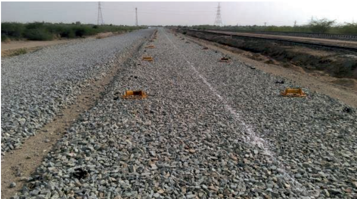
Fig. 7.11 Centre Line of Alignment Marked.
