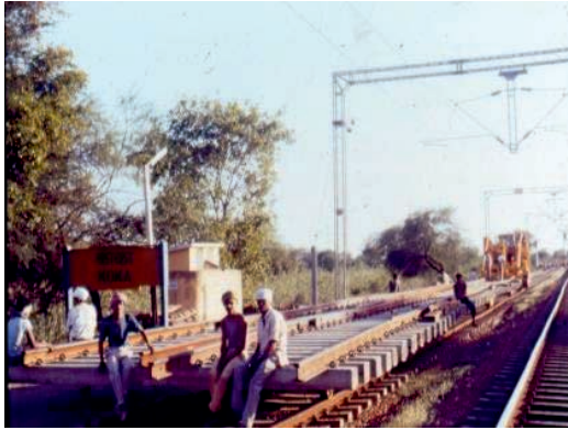
Fig. 6.7 Fabricated Panel on Trolleys being Toed
