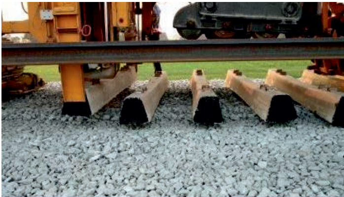
Fig. 7.19 Laying of Sleepers at Equal Spacing
