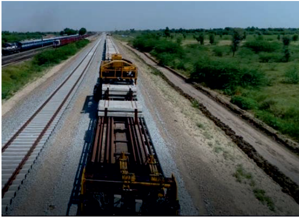
Fig. 7.14 Puller in M/s Harsco NTC Machine
