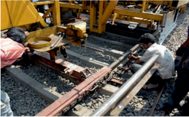
Fig. 5.3 Sled being Connected to Rail.
