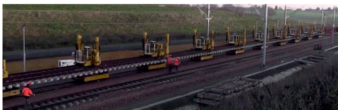
Fig. 10.2 (b) Giesmar Portal Carrying Prefabricated Panel
