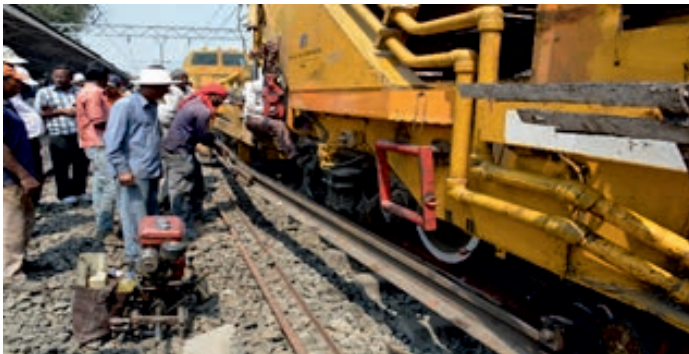
Fig. 5.6 Rail on One Side being Connected
