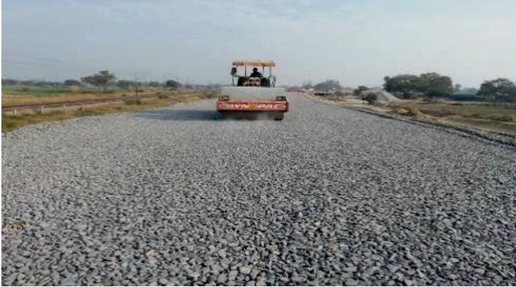
Fig. 7.10 The Ballast Bed is Laid in Advance.
