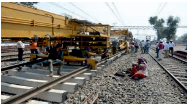
Fig. 5.11 Threading in Rail
