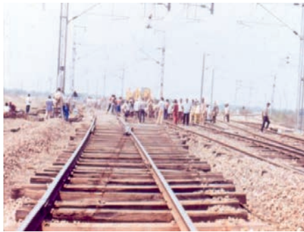
Fig. 6.13 Advance Dismantling of T/O Side Rails.
