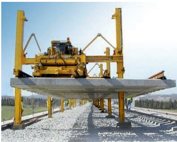
Fig. 10.2 (a) Giesmar Make Portal PEM and LEM used for Laying T/O and Plain Track also
