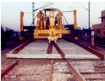
Fig. 6.9 Final Laying and Fixing New Panel to Track.
