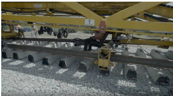
Fig. 7.20 Threading in of Rails behind NTC
