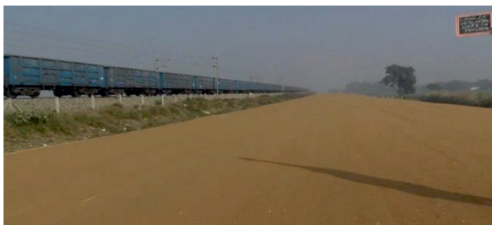
Fig. 7.8 Ready Formation for Laying of Ballast
