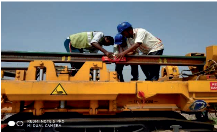
Fig. 7.15 Connecting Rails During Unloading.
